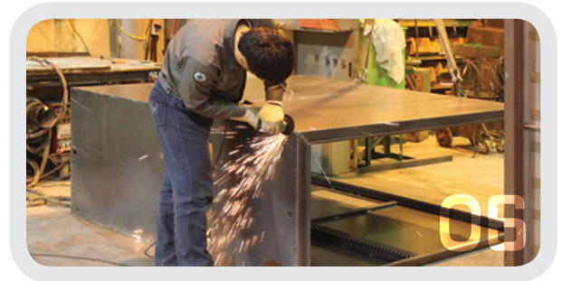
용접, 제관작업 (Welding, Piping Work)
